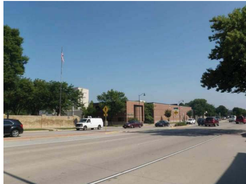
VIEW FROM EAST WASHINGTON LOOKING NORTHEAST
