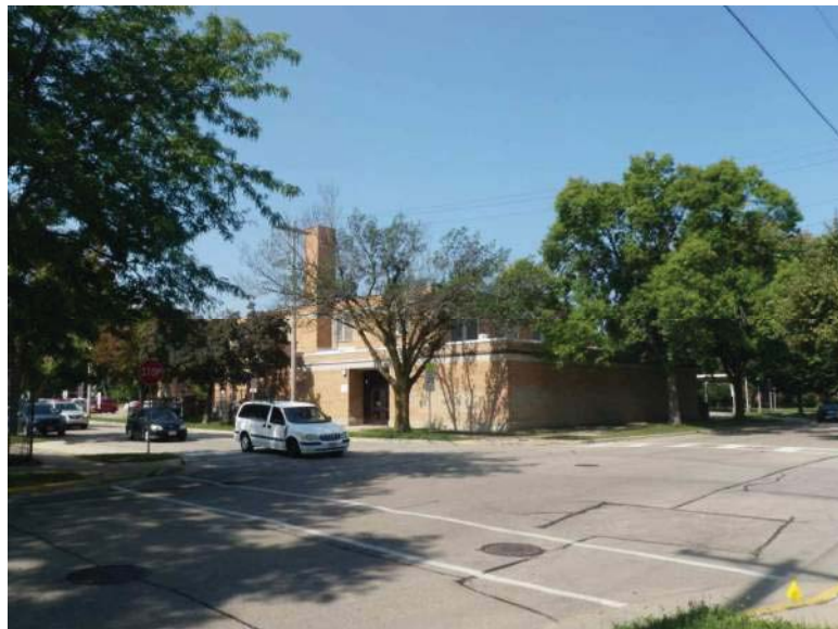
VIEW FROM MIFFLIN AND INGERSOLL LOOKING WEST
