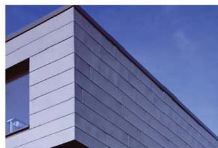
FLAT-LOCK STANDING SEAM METAL PANEL
