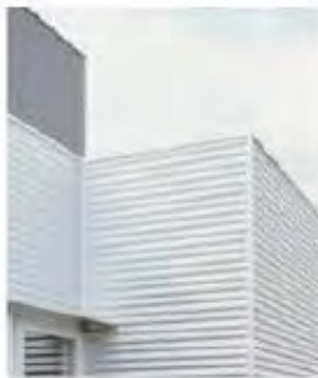
CORRUGATED METAL PANEL CONCEALED FASTENERS
